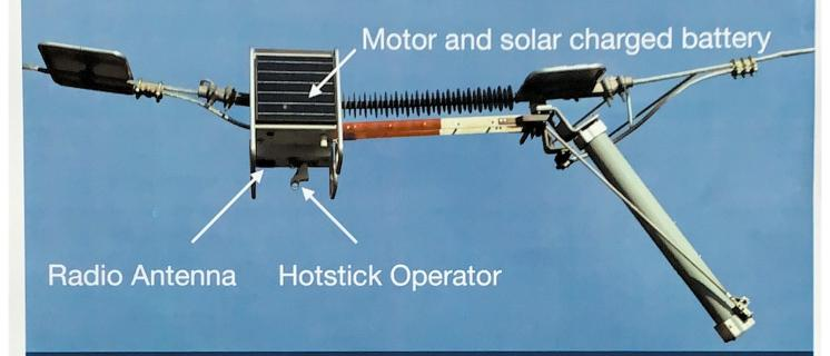
AutoLine®: No structure, no interphase linkage to adjust, and cuts in anywhere.
